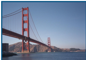
Golden Gate Bridge, San Francisco
